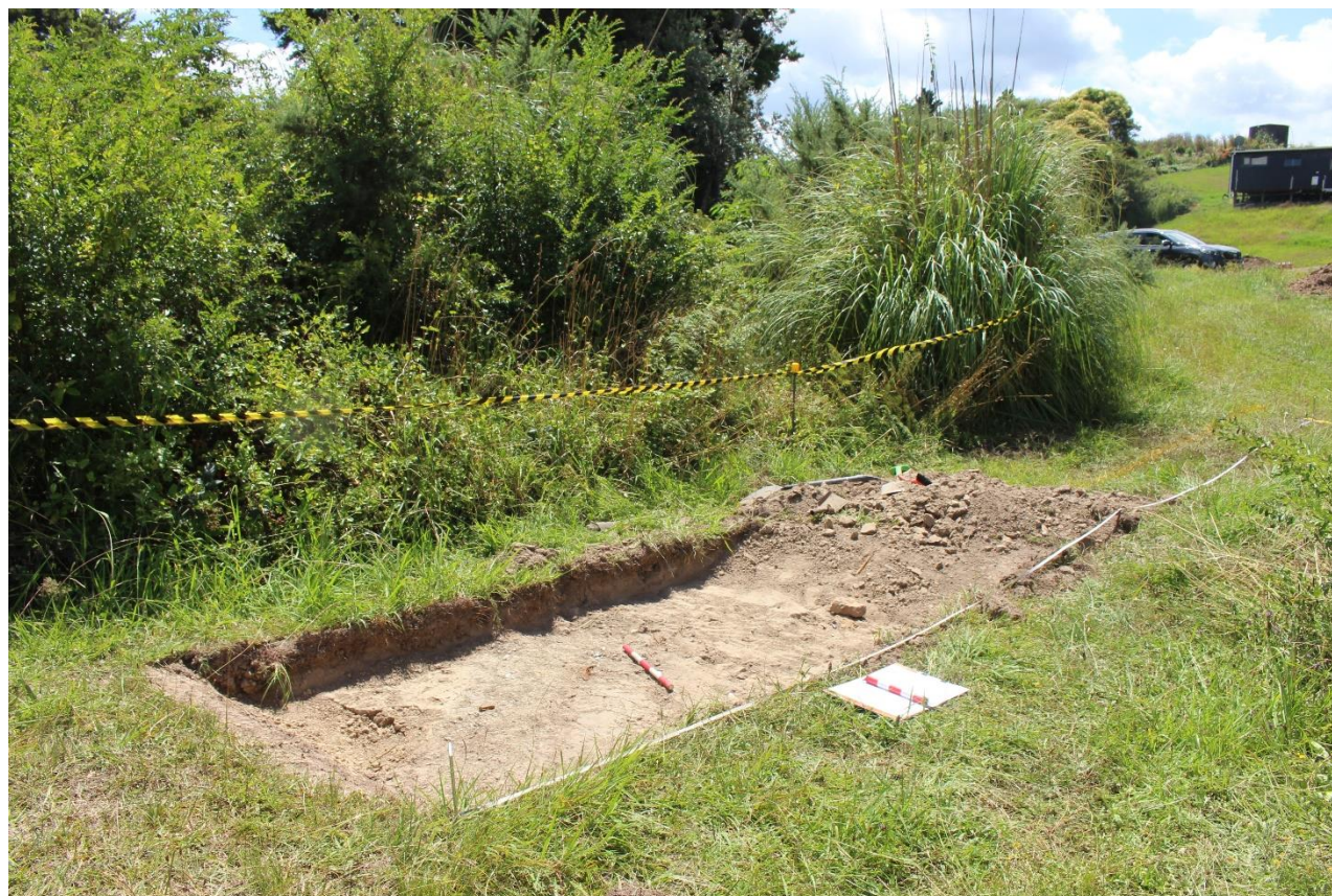
Site protection examples – protection of archaeological deposits (T06) with polypropylene geotextile cloth prior to backfilling as per HHMP. Hazard barrier tape demarcating 'no-travel' zones
