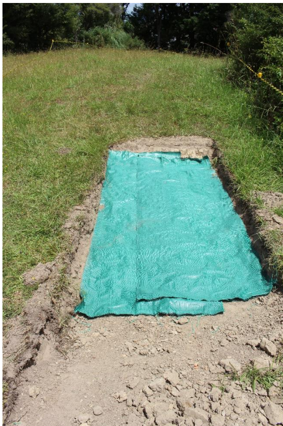
Site protection examples – protection of archaeological deposits (T06) with polypropylene geotextile cloth prior to backfilling as per HHMP. Hazard barrier tape demarcating 'no-travel' zones
